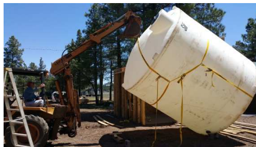
One of the 10,000 gallon water tanks being moved into position
