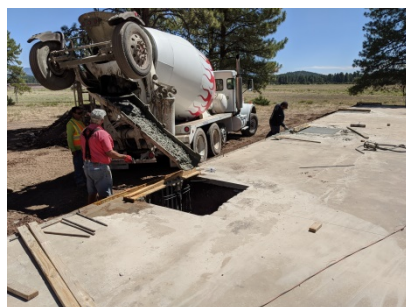
Concrete Piers for Steel Pillars
