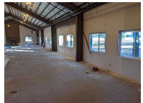
Drywall installation in auditorium
