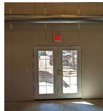
Exit signs and duct work completed
